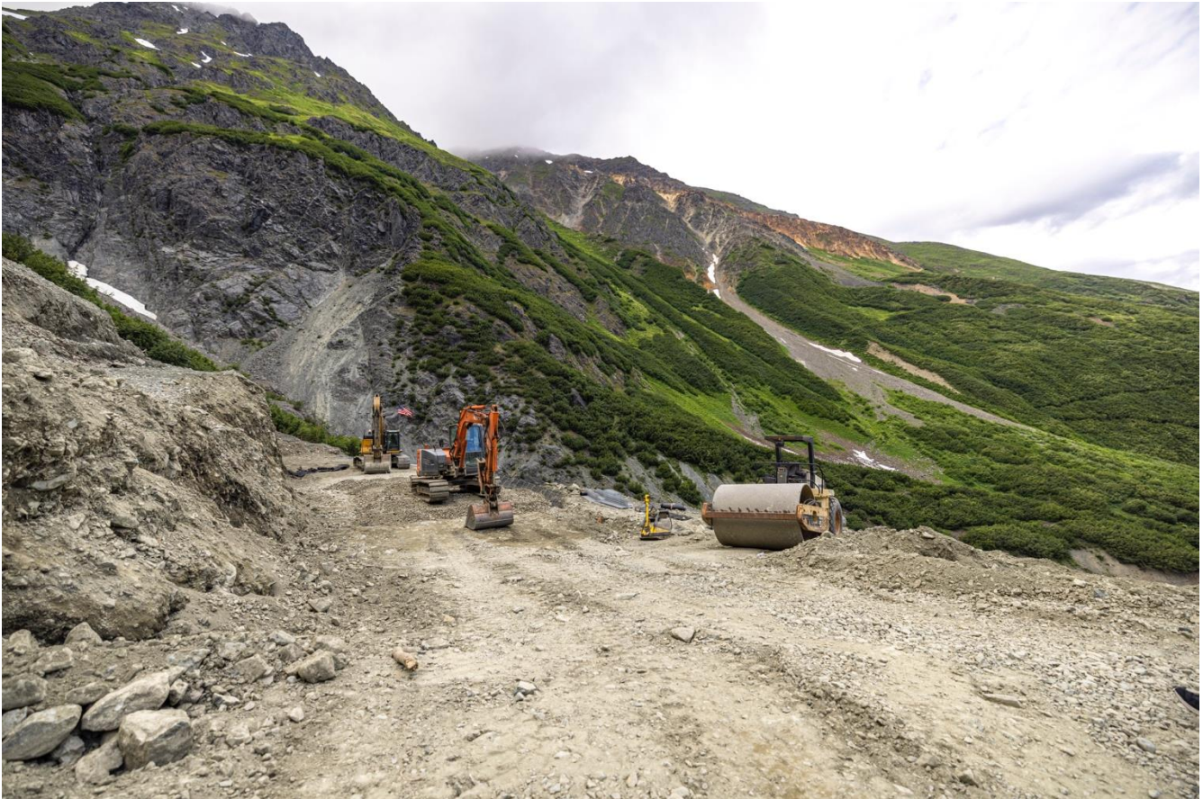
Image 1. Portal Access Road Construction
